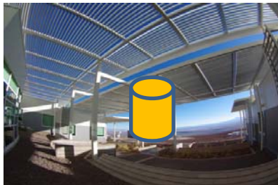
OSF (Operations Support Facility) @ 2900m
